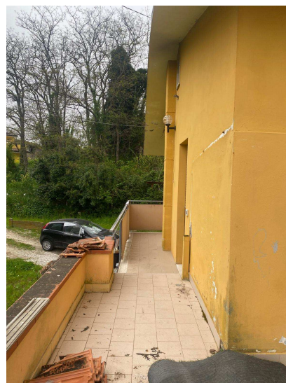
Balcone sub 3 PP
